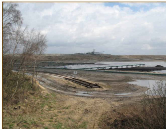
Fig. 2. Examples of by-products of energy production from coal in the Sokolov region: in the foreground ash-slag deposits of the Vřesová power station, in the background Smolnická spoil heap, where spoil substrate from the layers above the coal are deposited during mining. (O. Mudrák)
